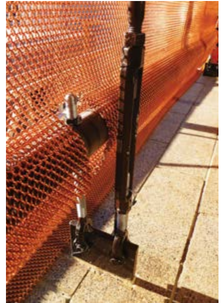
Antoine Predock Architect Studio chose coiled-wire fabric for a multi-panel assembly at the U.S. Courthouse in El Paso, Texas.
