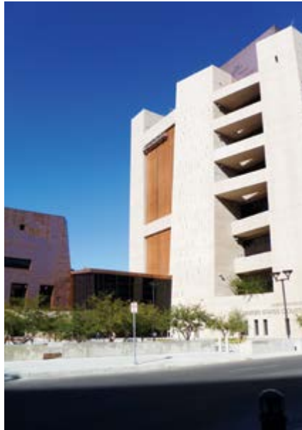
Antoine Predock Architect Studio chose coiled-wire fabric for a multi-panel assembly at the U.S. Courthouse in El Paso, Texas.
