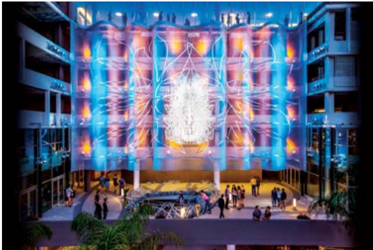
Also shown on page 18, the Vermont multi-family/retail complex uses a coiled-wire fabric system in an undulating profile as both the façade to its parking garage and as the canvas for Cliff Garten Studio’s art piece, “Los Angeles Opens its Heart of Compassion.”
